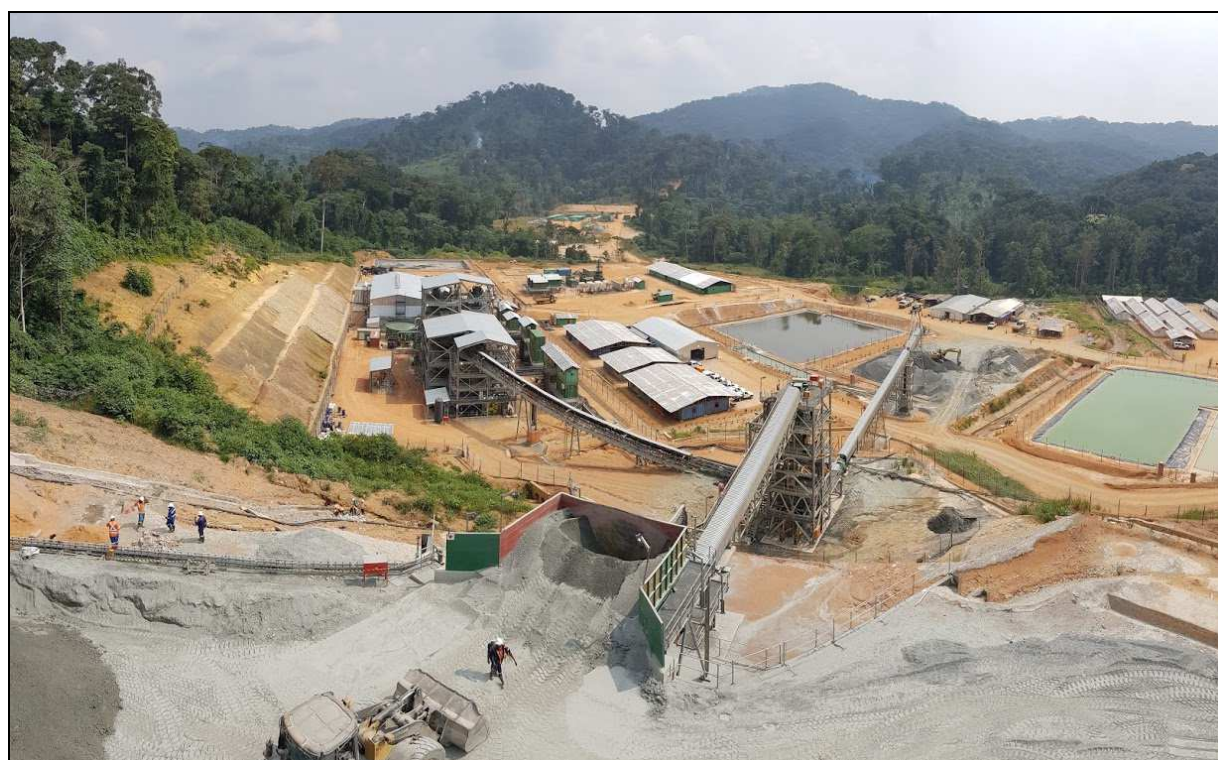
Crushed ore stockpile above jigs, gravity building to the upper left
